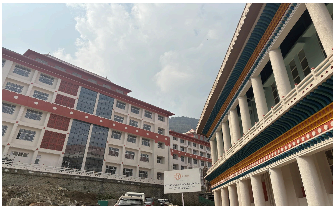
(Upcoming Sikkim University Campus at Yangang, South Sikkim)
