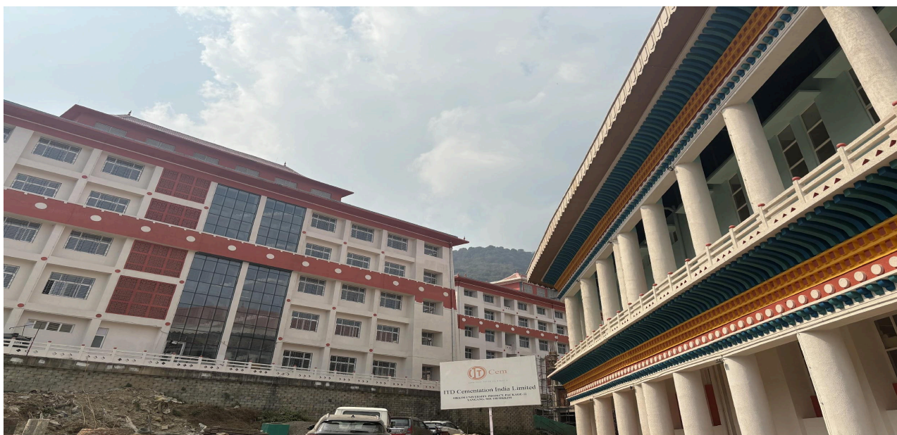
University Campus at Yangang, South Sikkim
