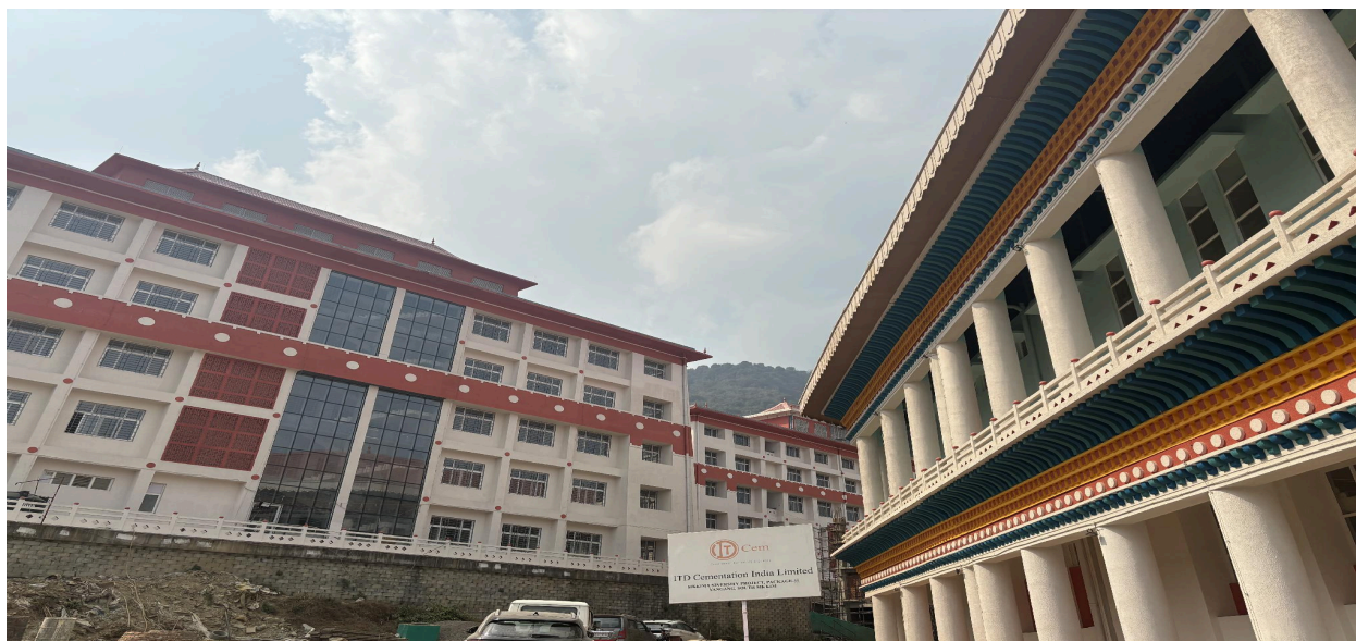
(Upcoming Sikkim University Campus at Yangang, South Sikkim)
