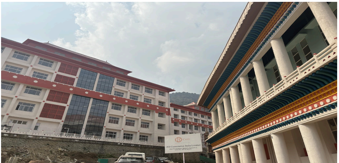
University Campus at Yangang, South Sikkim
